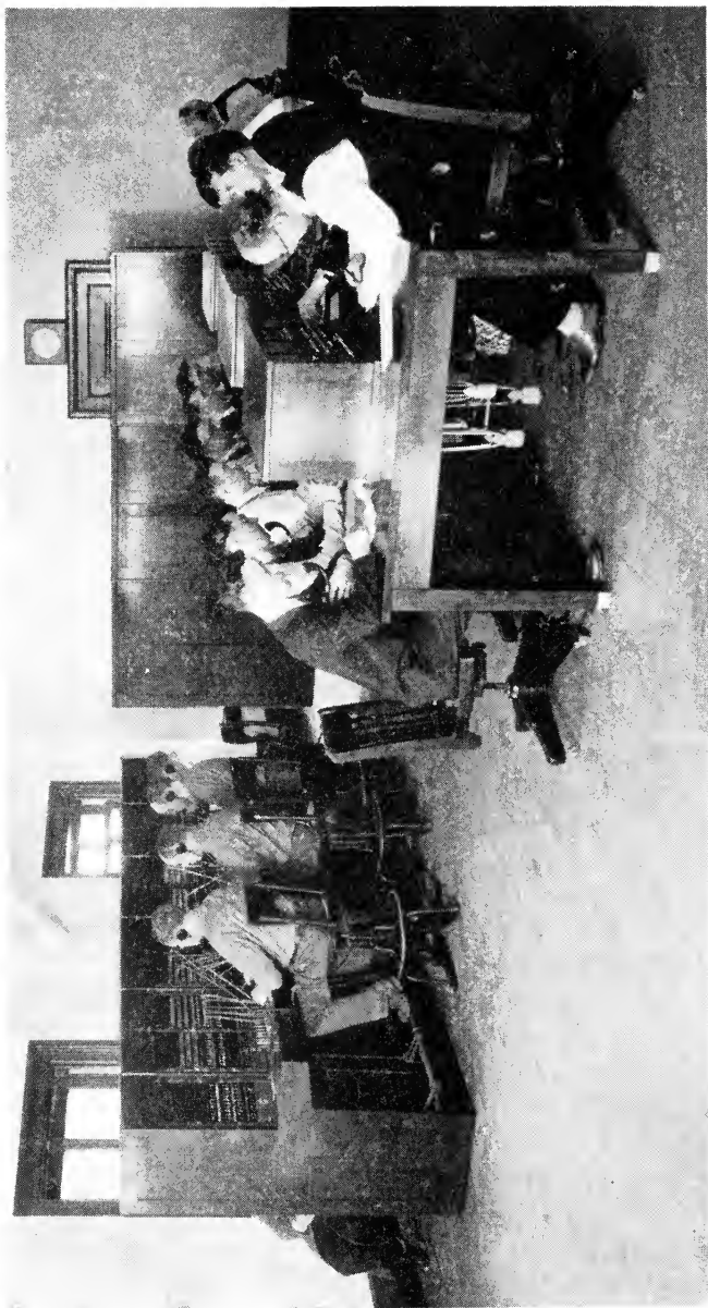
Telephone room at New York City police headquarters. At left, switchboard used for administrative calls; at right, receiving turret for emergency calls. The two are connected, so that calls coming to one may be transferred without delay to the other.
